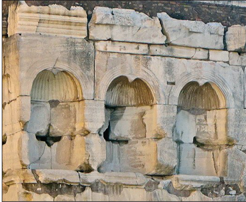
Figure 2. One row showing the scalloped crowning of the niches of the Arch of Janus.
