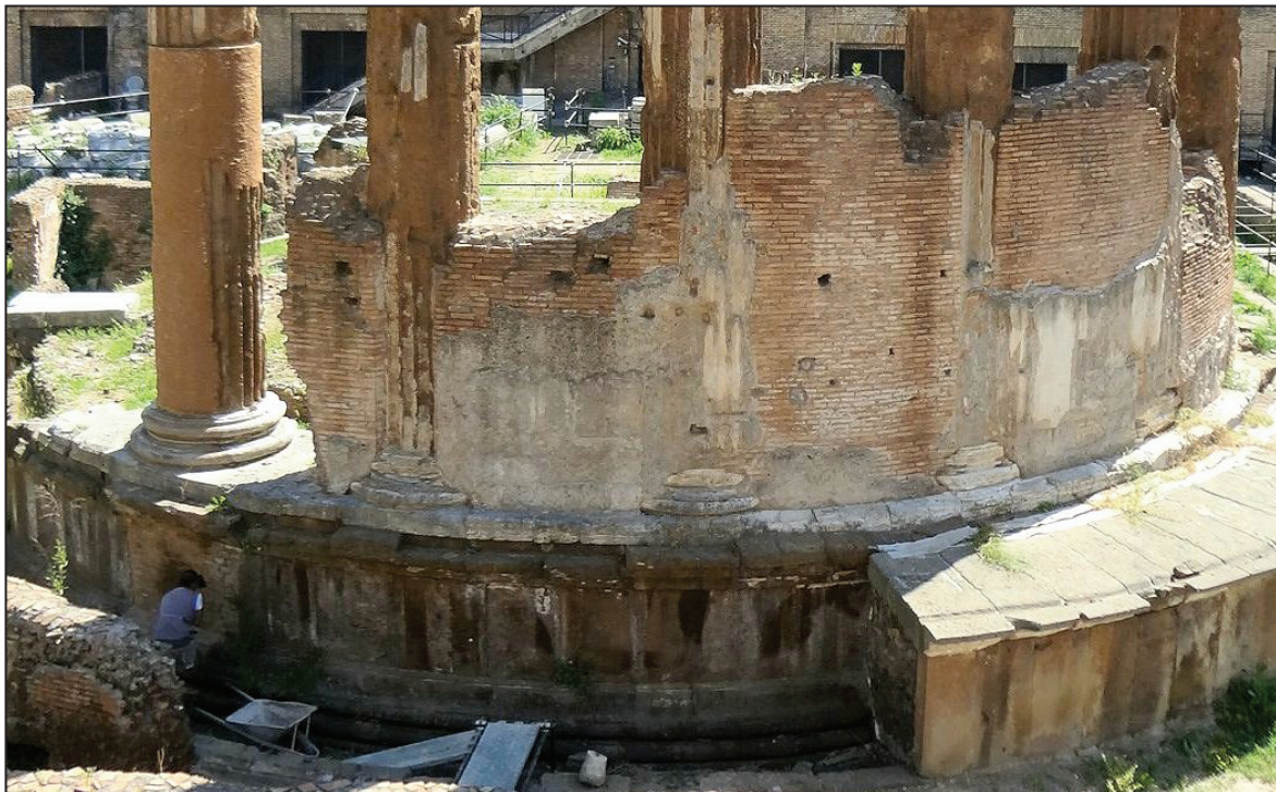
Figure 7. The restorations after the fire of 80 A.D. can be seen in the photo of Temple B. The central cella of the temple was removed and the space between the columns was filled in with a brick wall. That wall was then faced with brick so that the columns could not be seen. (Photo: Louis F. Aulbach)
