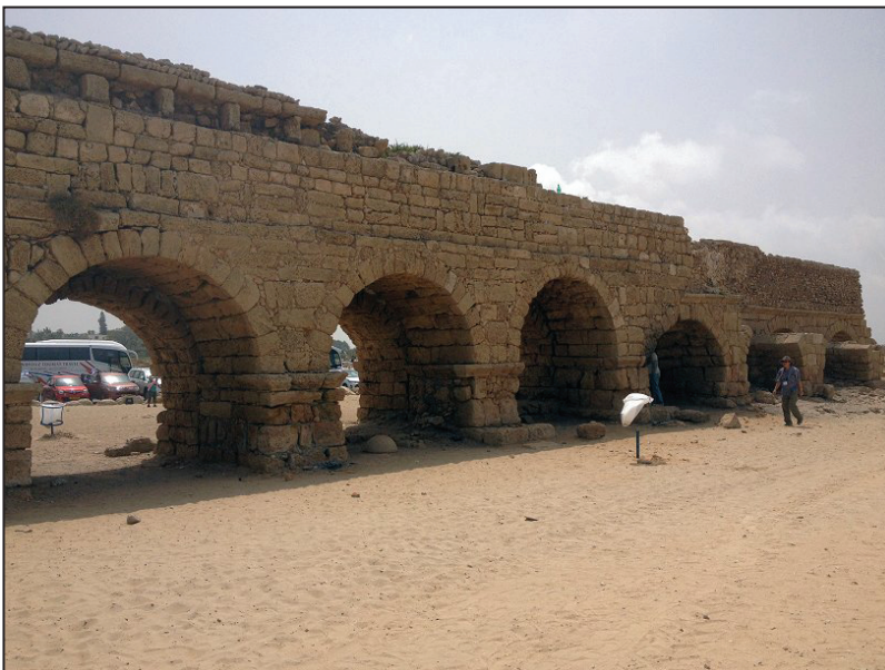
Figure 3. Detail of the major aqueduct system at Caesarea, Israel in which you can clearly see the two structures side-by-side within the arches.
