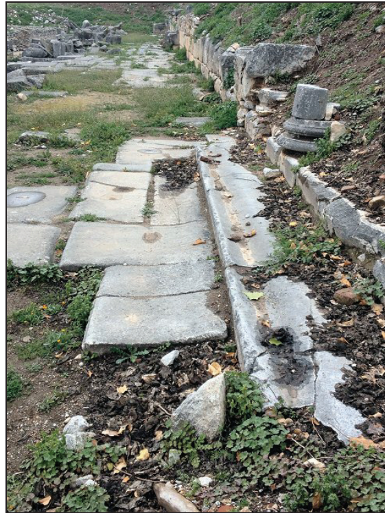
Figure 4. Detail of the Via Egnatia at Philippi showing gutter system.
