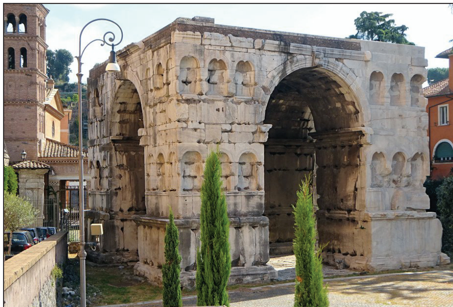
Figure 1. The Arch of Janus is constructed of brick-faced rubble clad in marble. Rows of niches cover the exterior surface of the piers. (Photo: Louis F. Aulbach).
